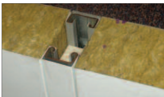
Figure 17: Insulated core panels – internal panel
